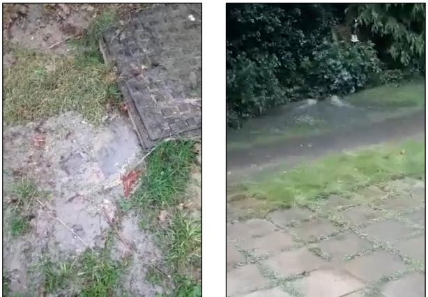
Frame grabs from cell phone videos of two separate incidents. On the left sewage is erupting from close to an inspection chamber. On the right sewage is gushing out with some considerable force from the underground sewage main.
