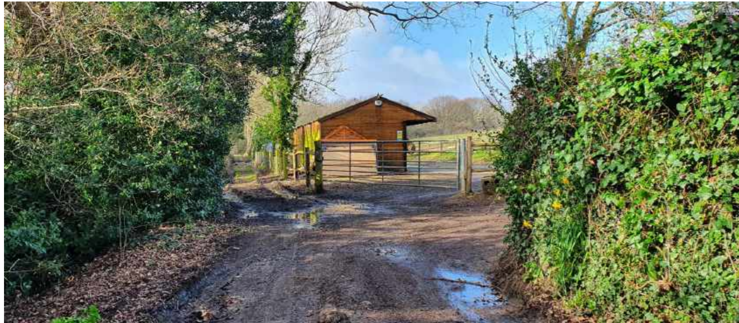
View of existing stable building from pedestrian footpath looking south west
