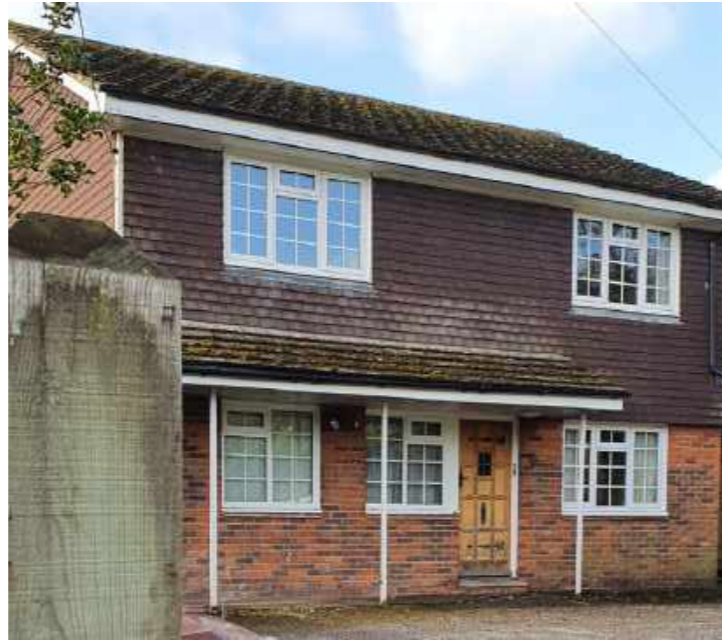
Existing dwelling to be demolished to create entrance
