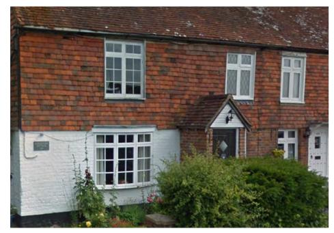
Brick painted white on the ground floor and clay hung cladding on upper floor
